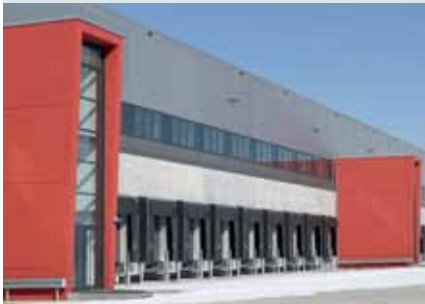
Immogate Logistikcenter, München
